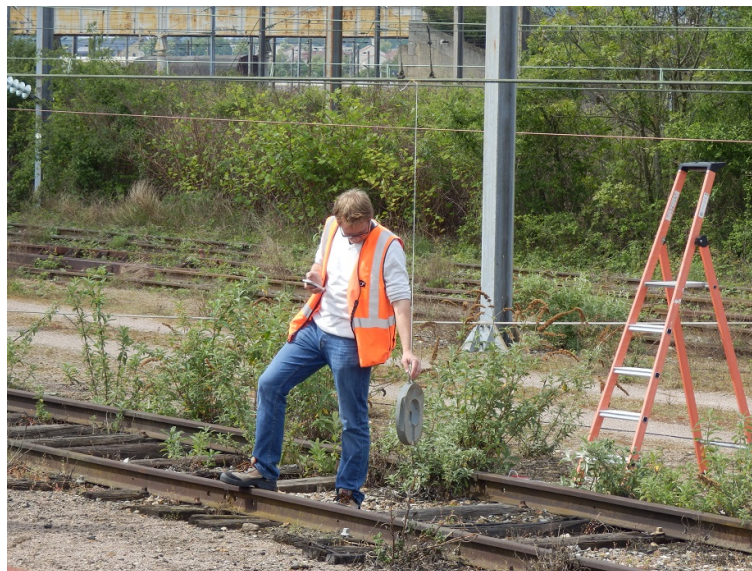
Figure 1.22: A mass drop test on the full size catenary
